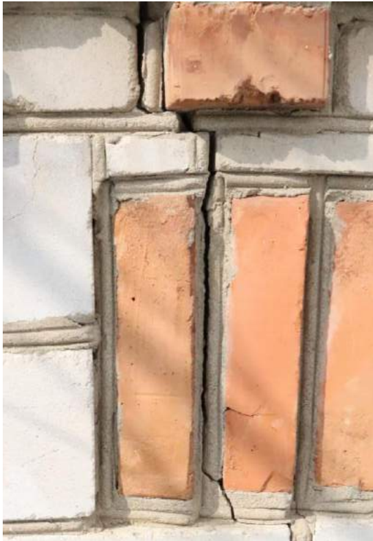
Cracks have appeared in recent years in residents' homes close to the road, both on building exteriors and along the walls and ceilings of interior rooms.
